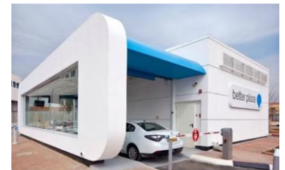
A Better Place switching station in Israel around 2012
