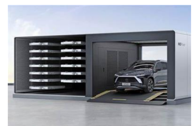
This is a Nio battery changing station with the changing bay and adjacent battery storage room. It has thirteen batteries and one open slot for the battery that is taken out of the vehicle
