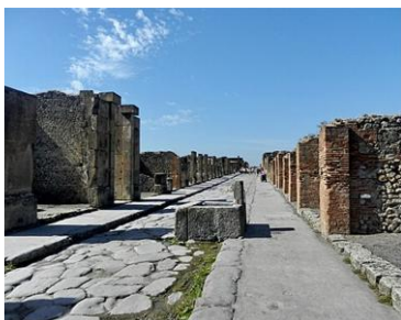
Raised sidewalk called samita ('footpath') with stone curbs beside a Viae vicinales in Pompeii, Italy
