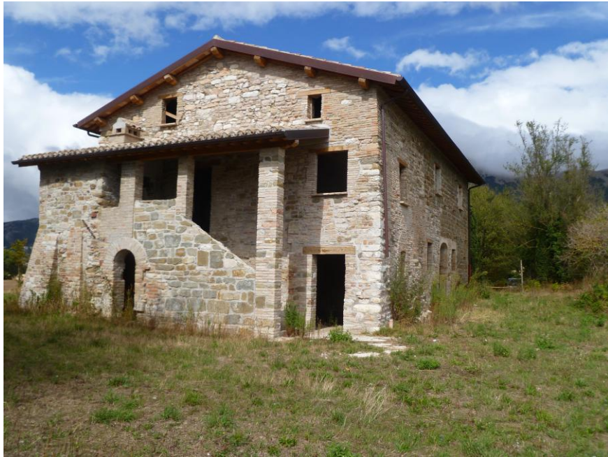
Masseggio under renovation - 2012
