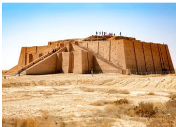
The ziggurat at Ur was built during the reign of King Ur-Nammu (2112–2095 B.C.).
